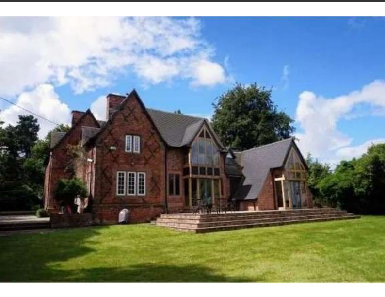
The project included the installation of **over 12,000 Staffordshire Blue 10x6 tiles**, over 80 collared ridge tiles, 32 linear metres of mortar gable verges, and 21 linear metres of secret valleys (closed cut). Additional work involved a tiled dormer cheek with 17m lead aprons and 12m step flashings, along with a turret featuring lead over rolled hip timbers.
